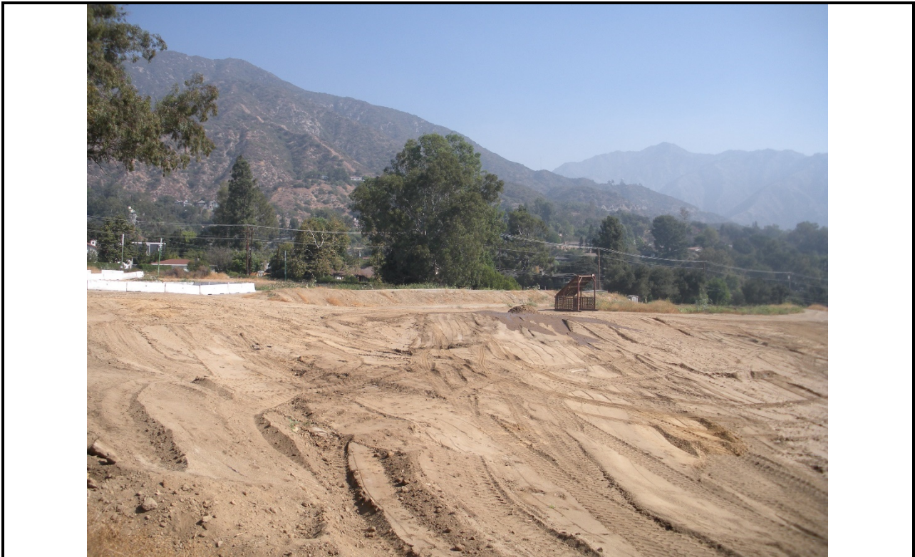
Photo 4. North-northeast view from southwest area (soil/rock screener in background).
