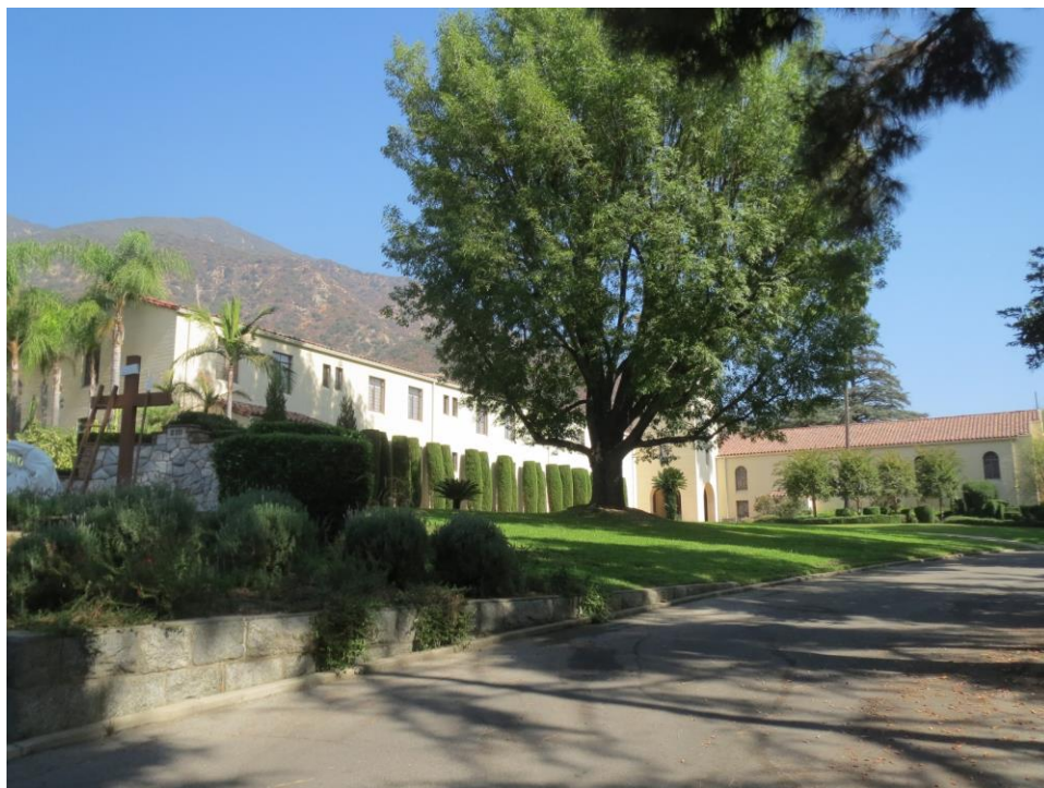
Figure 14. Retreat Center building: South and west elevation of 1951 original building and chapel, looking northeast (IMG_4868)
