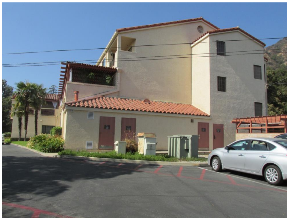
Figure 19. Retreat Center building: East and South Elevation (1985 addition), View looking west (IMG_0933)
