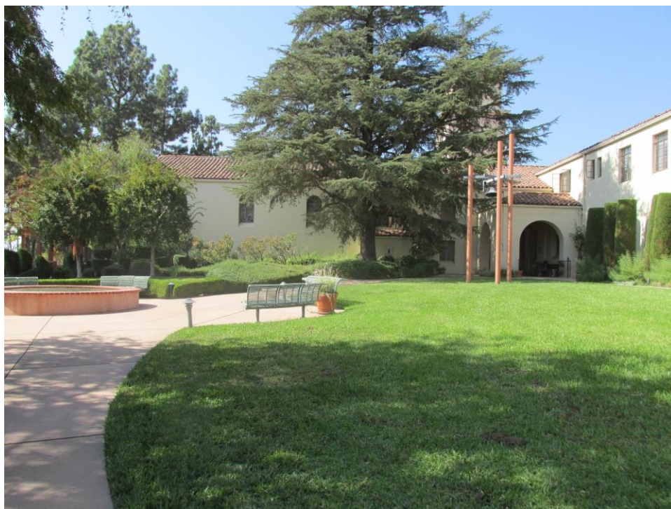
Figure 23. Retreat Center Chapel: East Elevation, View looking west (IMG_0977)
