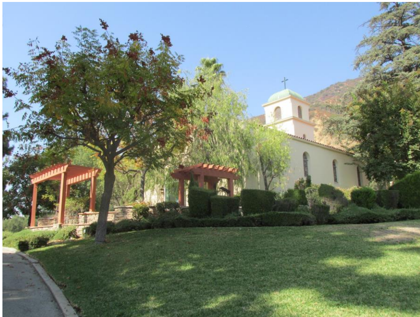
Figure 1. Retreat Center Chapel: East Elevation and South Elevation, view looking northwest (IMG_1022)
