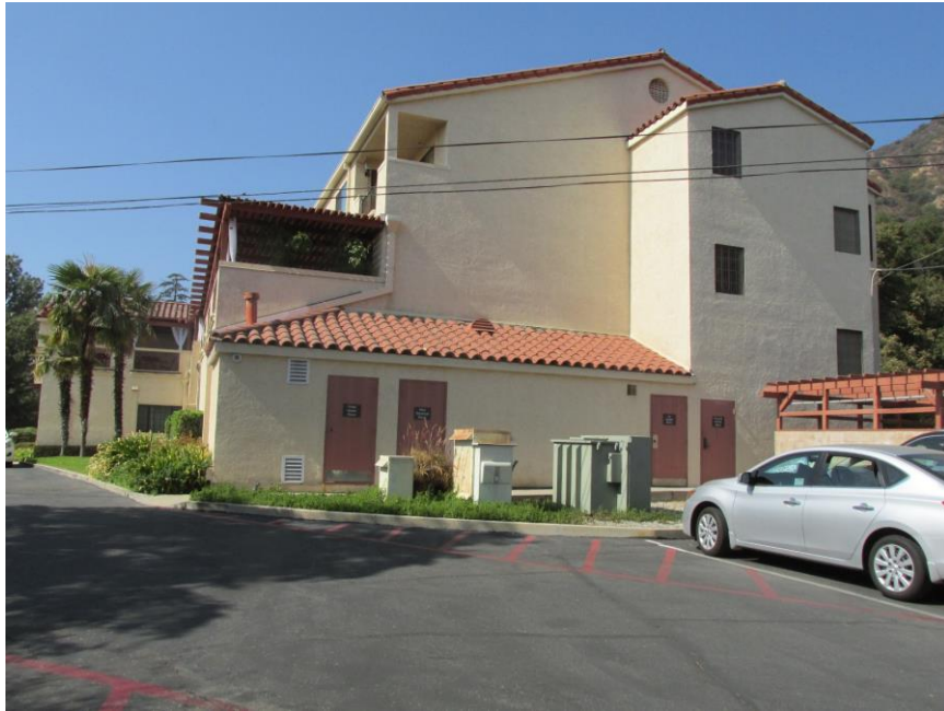
Figure 10. Retreat Center building: East and South Elevation (1985 addition), View looking west (IMG_0933)
