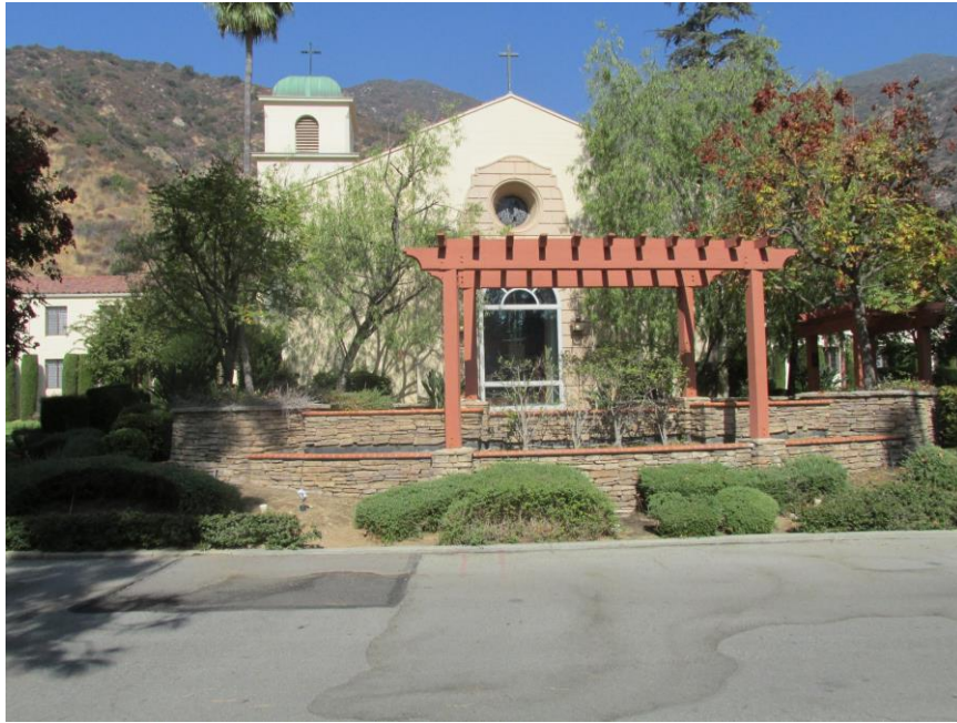
Figure 2. Retreat Center Chapel: South Elevation, view looking north (IMG_1027)
