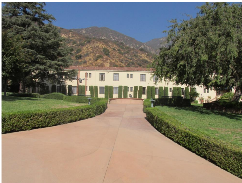
Figure 22. Retreat Center building: South Elevation, View looking north (IMG_1021)
