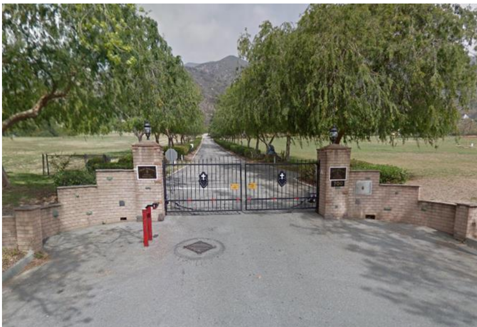
Figure 39. Sunnyside Avenue gate, looking north (Google Earth)
