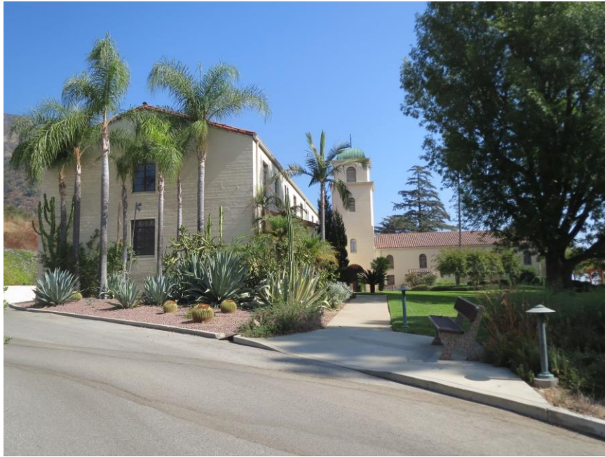
Figure 6. Retreat Center building: West Elevation, View looking east (IMG_4874)
