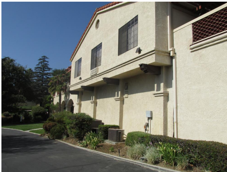
Figure 20. Retreat Center building: South Elevation (1985 addition), View looking northwest (IMG_0948)
