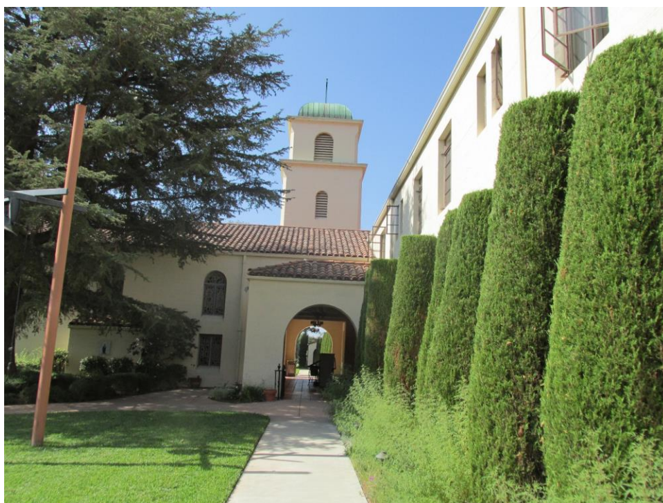
Figure 24. Retreat Center Chapel: East Elevation showing breezeway detail, View looking west (IMG_0991)
