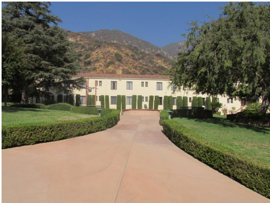
Figure 13. Retreat Center building: South Elevation, View looking north (IMG_1021)
