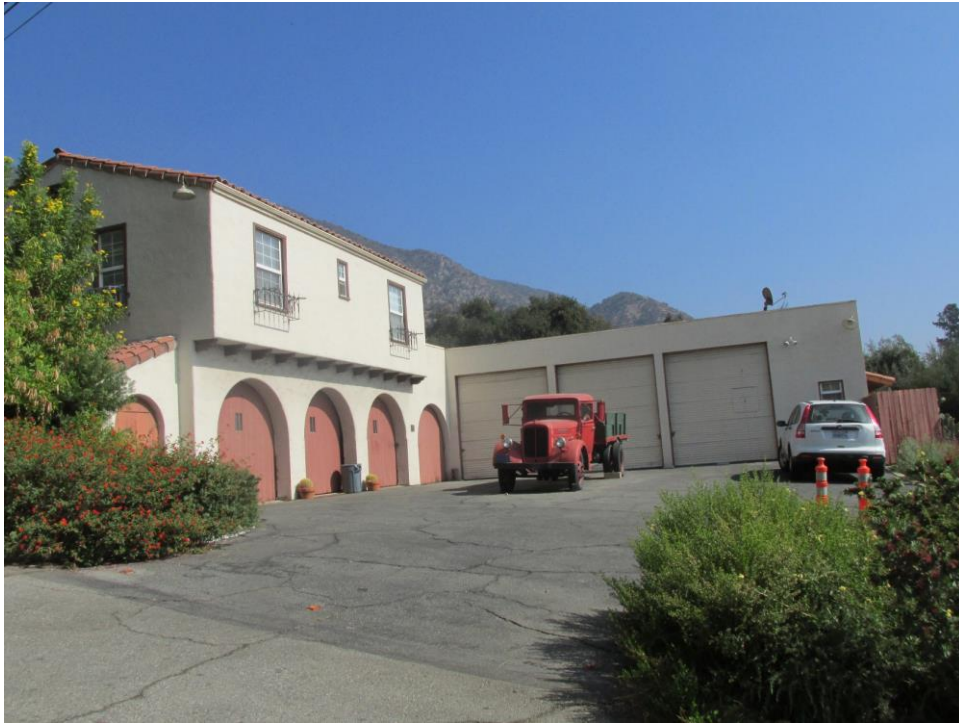
Figure 17. Building 1: West and south elevation, View looking northeast (IMG_0806)
