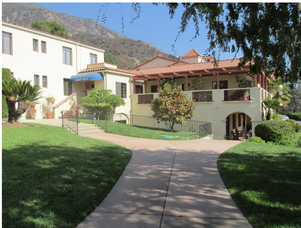
Figure 21. Retreat Center building: West and South Elevation (1985 addition), View looking east (IMG_0978)
