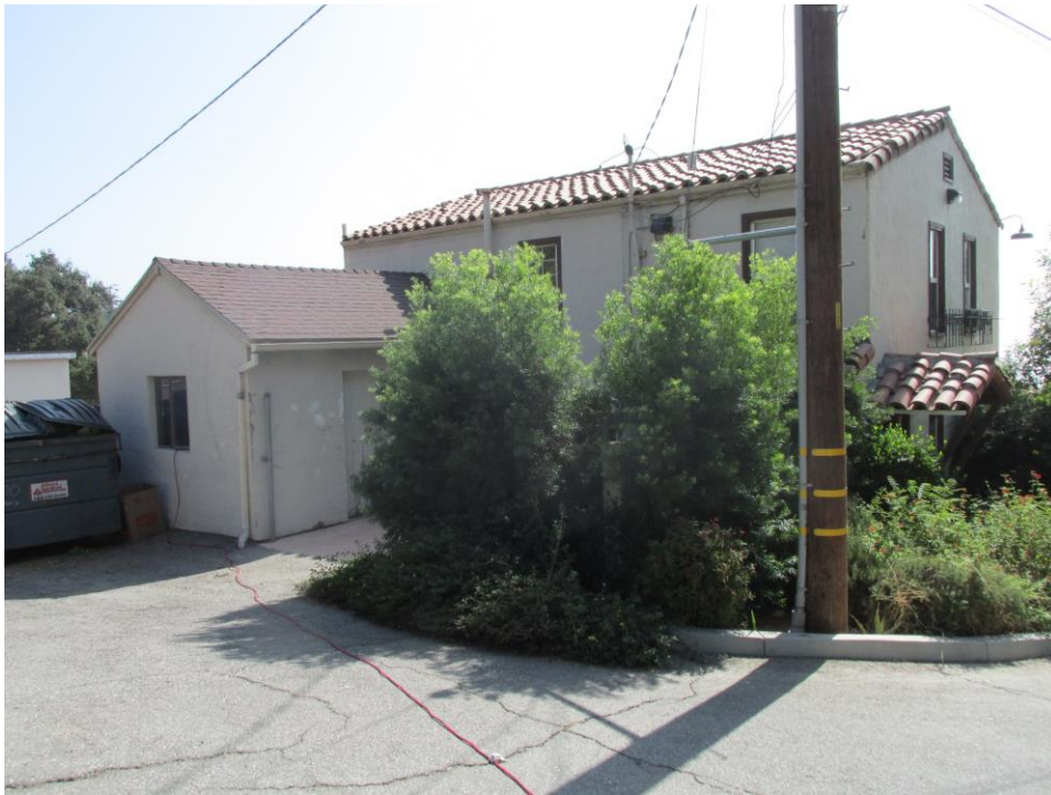
Figure 16. Staff House: North and west elevation, View looking southeast (IMG_0802)
