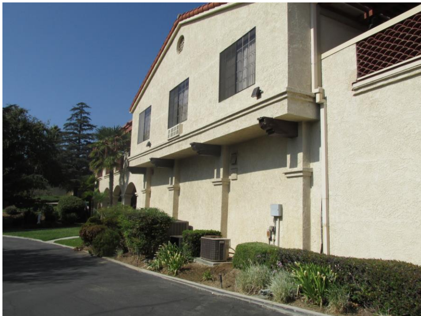
Figure 11. Retreat Center building: South Elevation (1985 addition), View looking northwest (IMG_0948)
