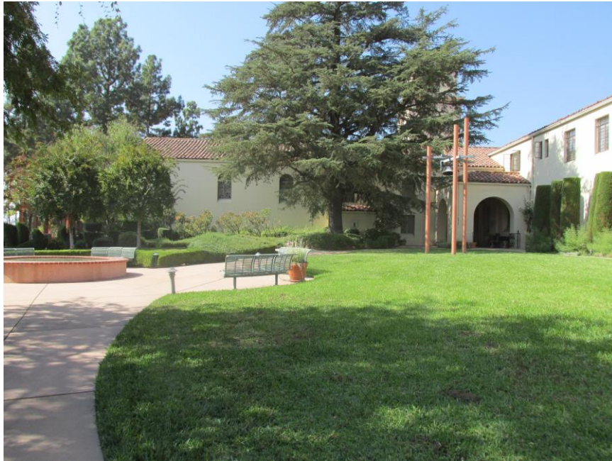
Figure 14. Retreat Center Chapel: East Elevation, View looking west (IMG_0977)
