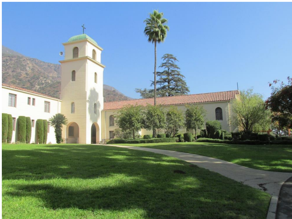
Figure 12. Retreat Center Chapel: West Elevation, view looking east (IMG_1041)
