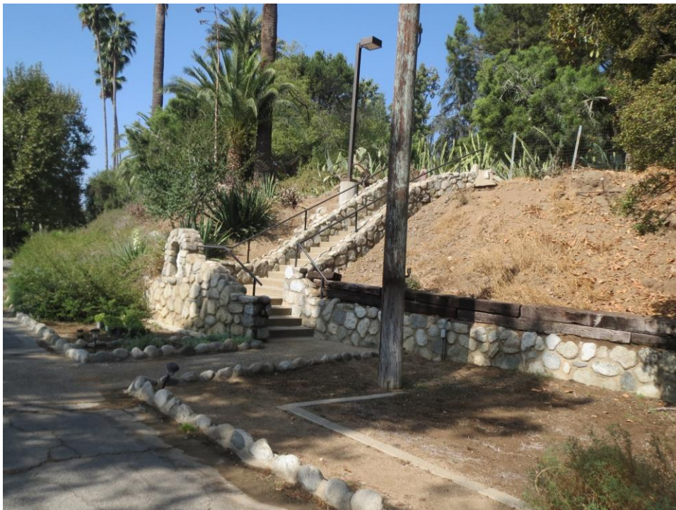
Figure 38. Example of typical stone retaining wall, stair and lined path. View looking northwest (IMG_4667)
