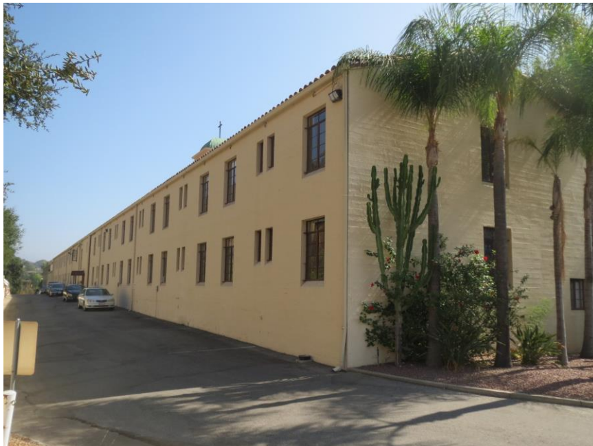
Figure 7. Retreat Center building: West and North Elevation, View looking southeast (IMG_4877)
