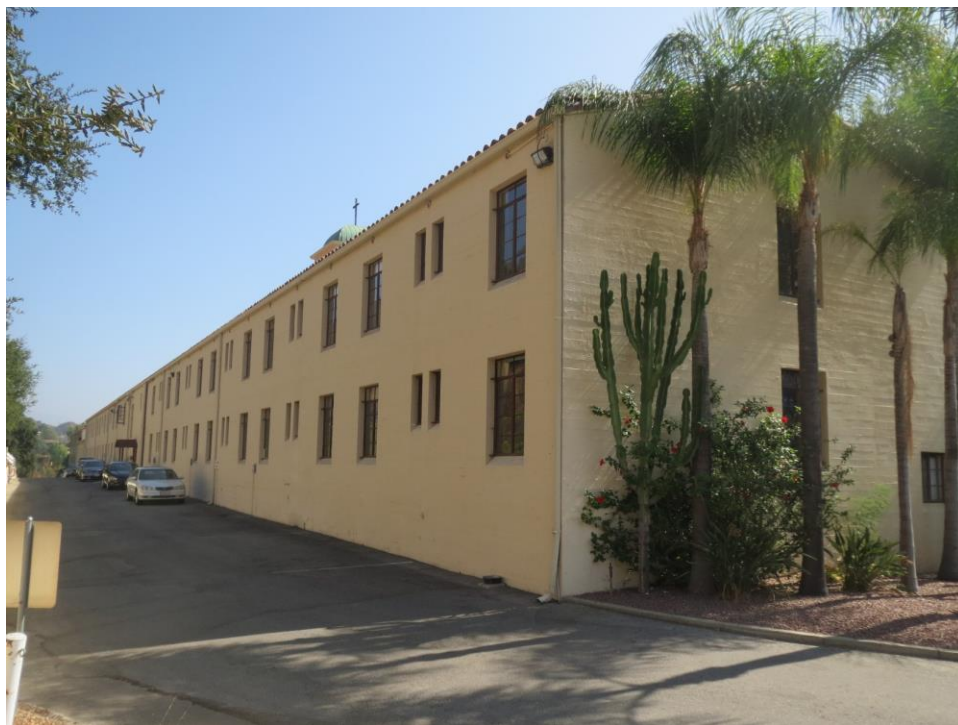
Figure 16. Retreat Center building: West and North Elevation, View looking southeast (IMG_4877)
