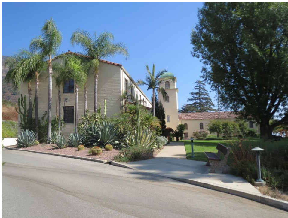
Figure 15. Retreat Center building: West Elevation, View looking east (IMG_4874)
