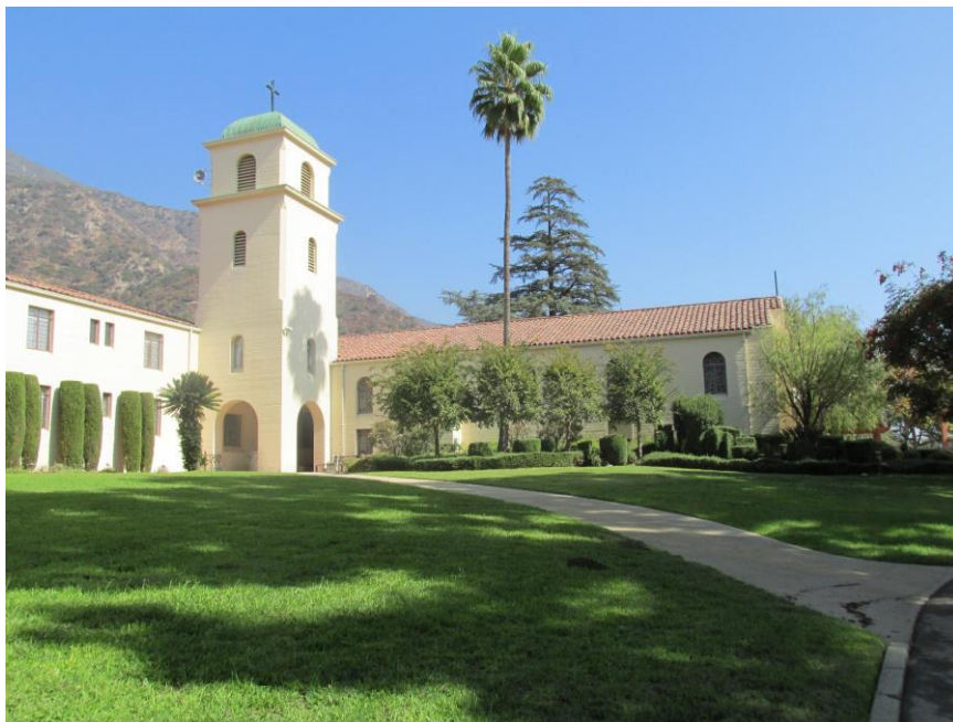
Figure 3. Retreat Center Chapel: West Elevation, view looking east (IMG_1041)
