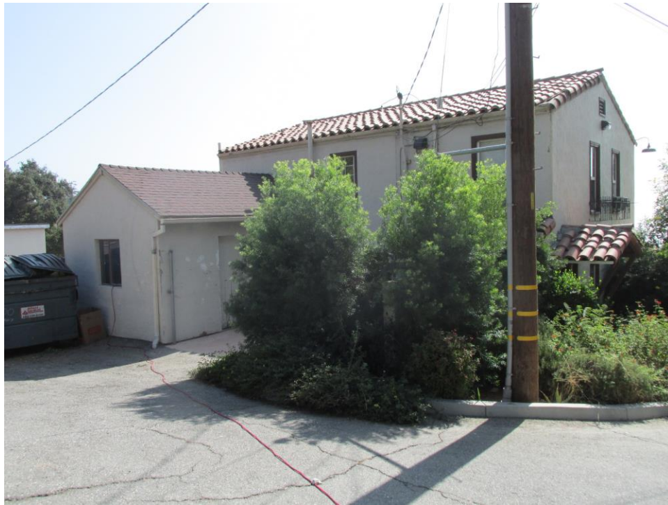
Figure 25. Staff House: North and west elevation, View looking southeast (IMG_0802)
