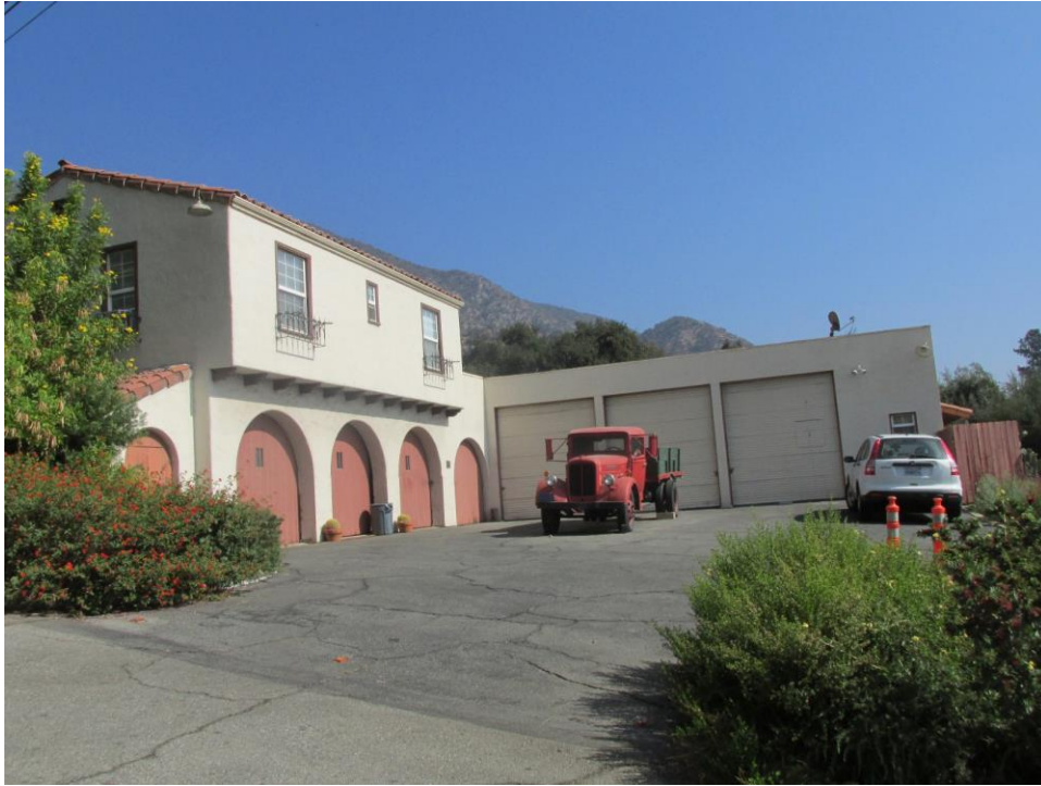
Figure 26. Building 1: West and south elevation, View looking northeast (IMG_0806)
