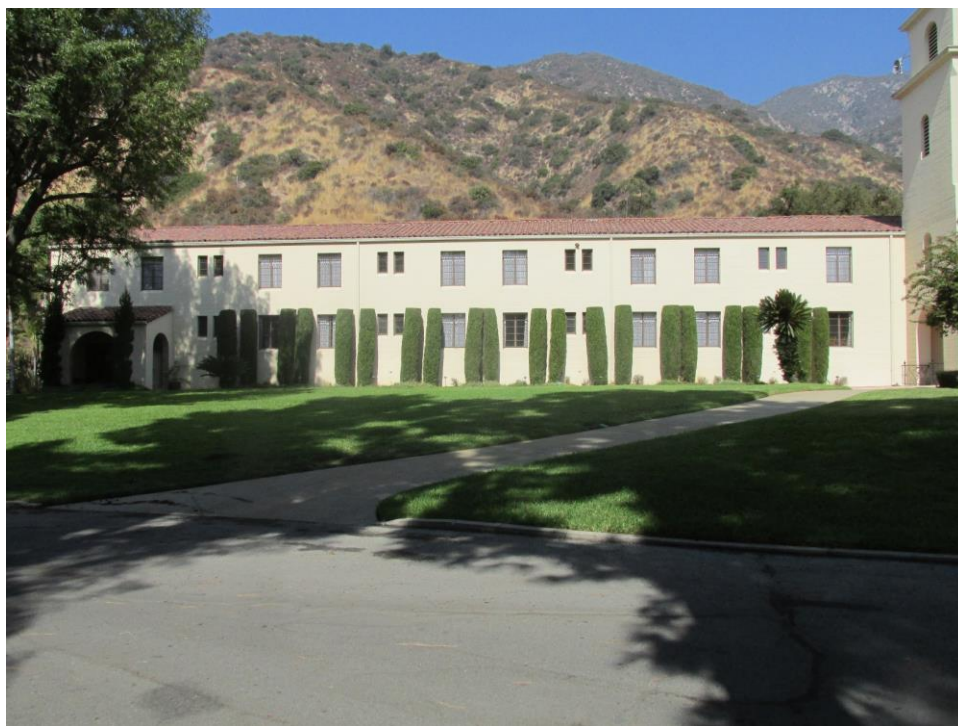
Figure 13. Retreat Center building: South Elevation, view looking north (IMG_1031)
