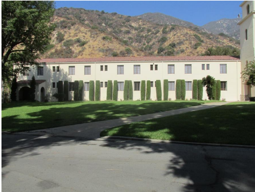
Figure 4. Retreat Center building: South Elevation, view looking north (IMG_1031)
