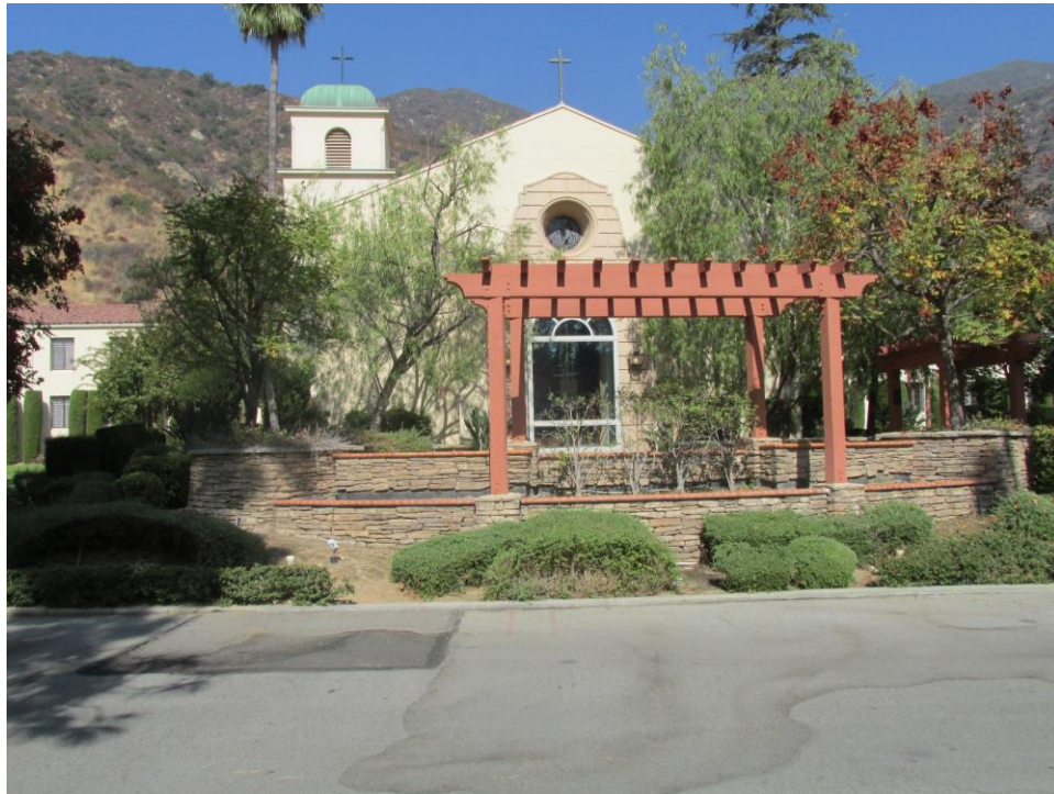
Figure 11. Retreat Center Chapel: South Elevation, view looking north (IMG_1027)
