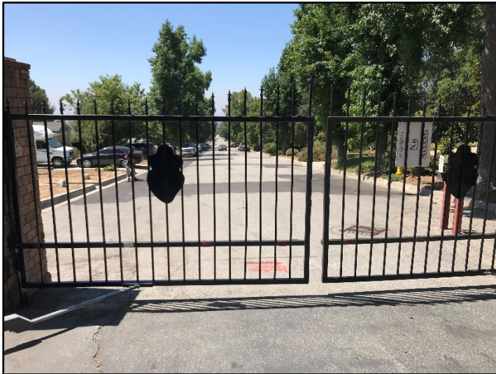
Photograph 3. View of gated roadway to the south along Sunnyside Avenue.
