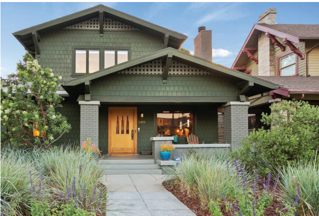
Appropriate: Articulated primary facade by stepping second stories back from the first.
