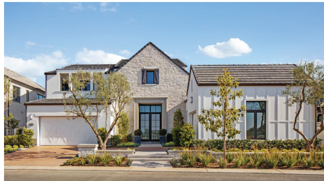
Appropriate: Building is oriented to and has visual connection with the street.
