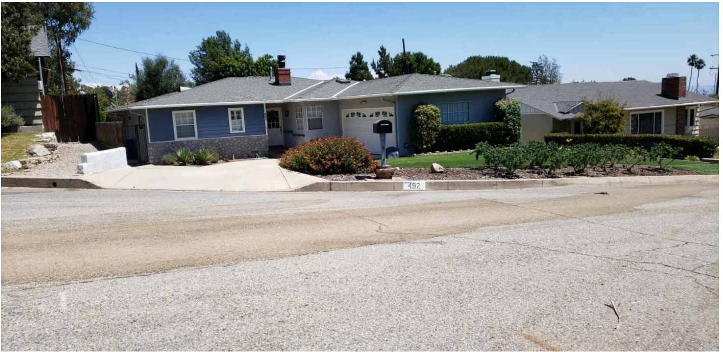
Water and Erosion Runoff at 492 Crestvale Drive. Flow pattern after the leak was repaired. 08/14/22.
