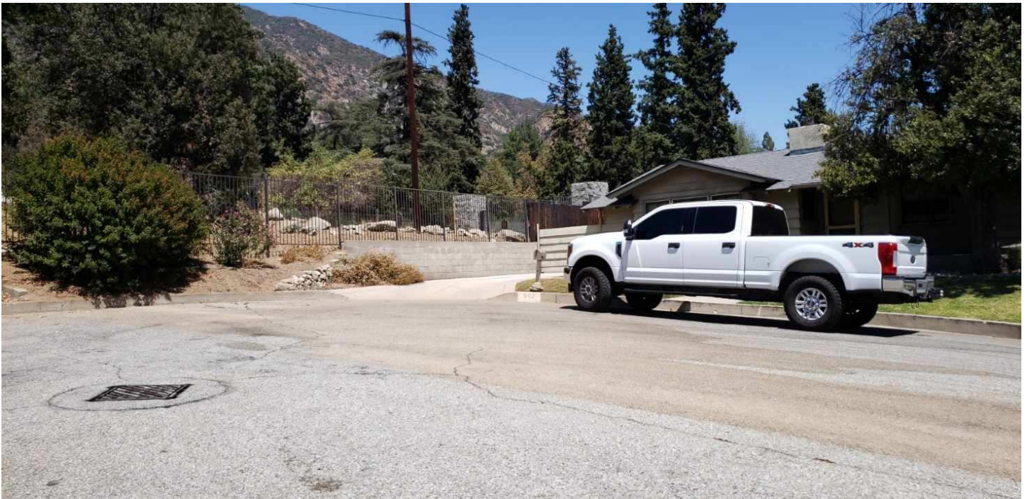
Water and Erosion Runoff at 502 Crestvale Drive. Flow pattern after the leak was repaired. 08/14/22.
