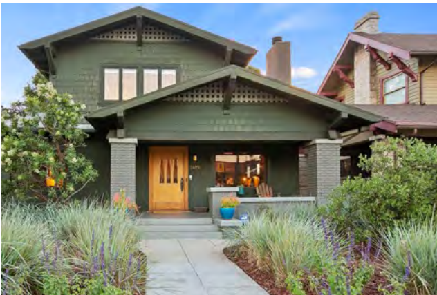
Appropriate: Articulated primary facade by stepping second stories back from the first.
