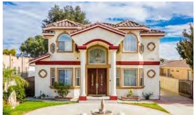
Inappropriate: Oversized, monumental primary door entry elements, e.g., two-story columns.
