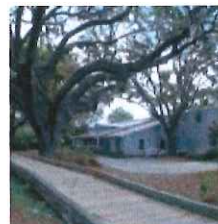
Bridging over tree roots can take many forms. This is an excellent example of a substantial bridge. But bridges do not have to be this large to protect roots. (Photo taken in Bluffton, SC)
