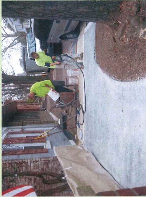
Trees Inc. covers its asphalt sidewalks with the same epoxy coating used in New York City.
