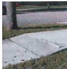
Three years prior to taking this photo, the lifted sidewalk slab had been replaced and the roots cut. In only three years the sidewalk had lifted again pushed up by new root growth. Cutting tree roots does not provide long term results and should be the last choice not the first.
