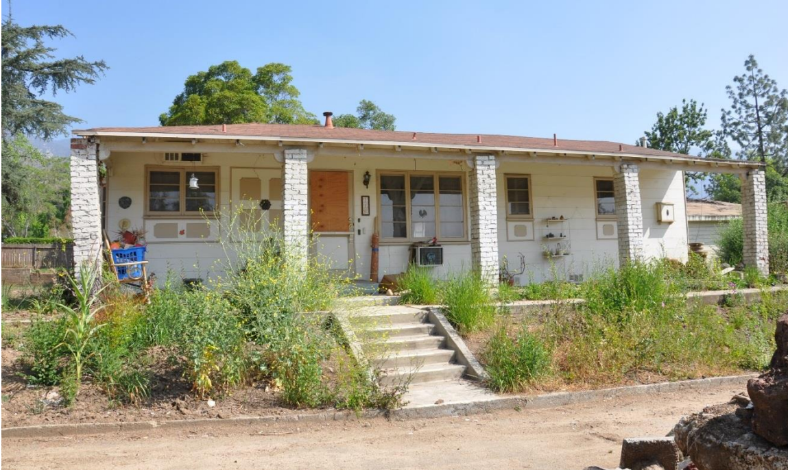
Figure 8. South façade of 110 Rancho Road with steps to the dirt driveway, looking north. Note the far left (north) and second from right (south) brick columns are out of plumb.
