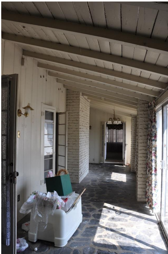
Figure 12: Enclosed rear (east) porch with original vertical wood siding and French doors.
